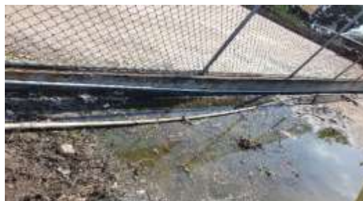
Figure 4. Wiring already distributed by the steel pipe
