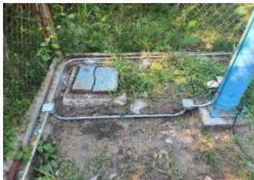
Figure 3. Steel boxes to be added to the pipeline for wiring
